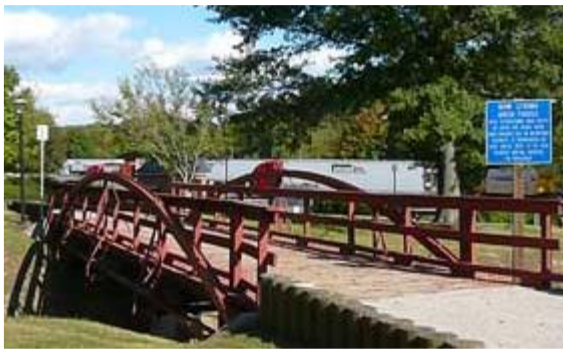
State's oldest metal bridge in Elliston
